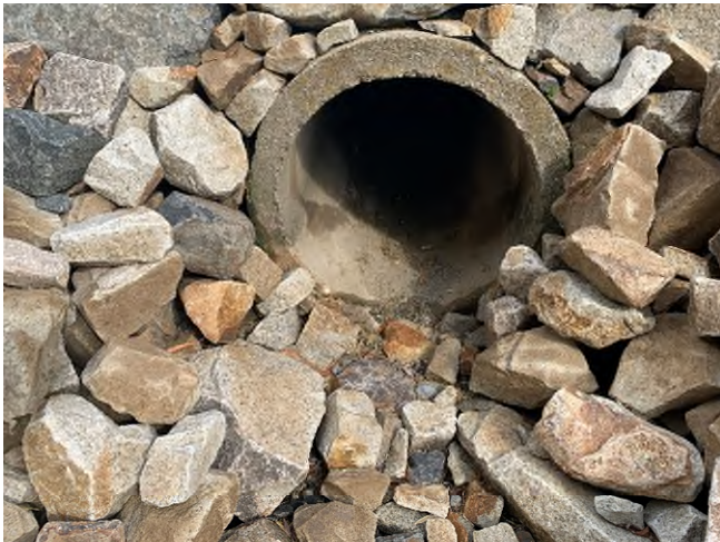
64 Gundalow - 1 (Drainage Course)
