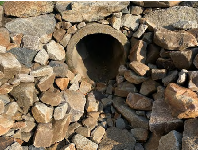
64 Gundalow - 1 (Drainage Course)
