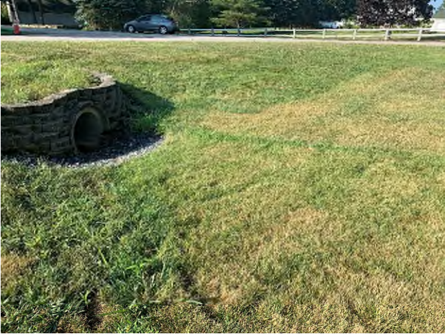
29 Gundalow - 1 (Drainage Area)
