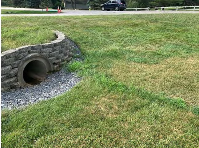
29 Gundalow - 1 (Drainage Area)
